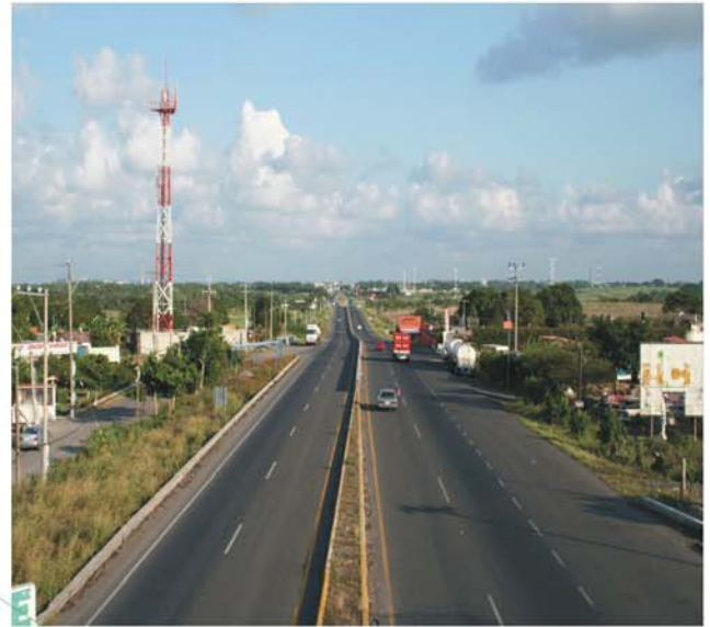
Carretera: Cardel - Tihuatlán, Ver.
